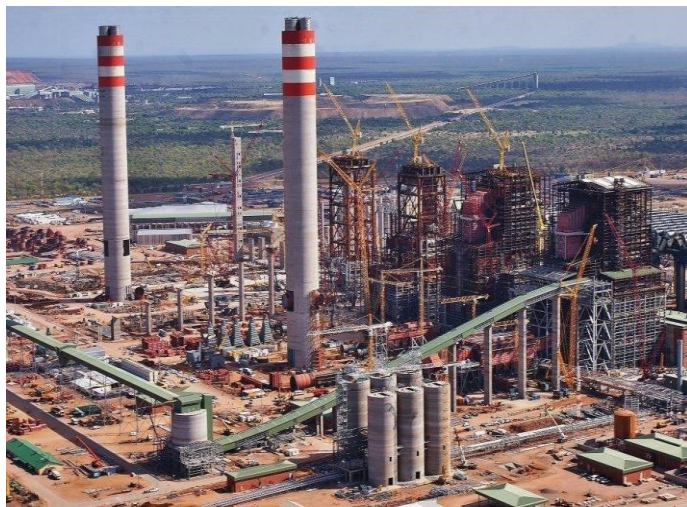
Kusile Power Station Construction
