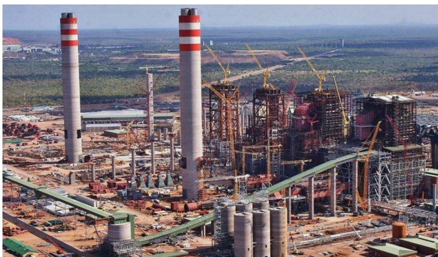
Kusile Power station construction.
